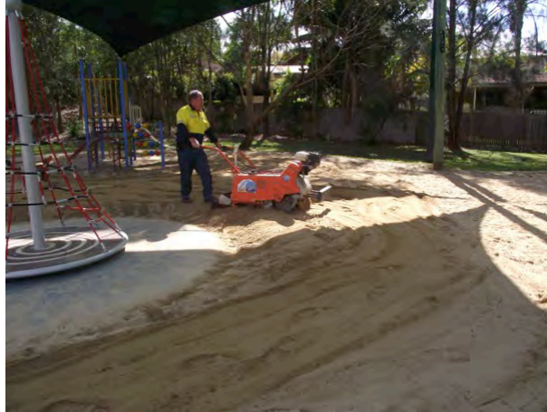
In-situ sieving using portable vibrating sieve
