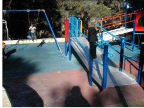
Figure 19: Ramp for access. Photo courtesy of Barbara Champion, PRAV
