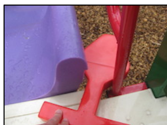
Examples of unacceptable openings
