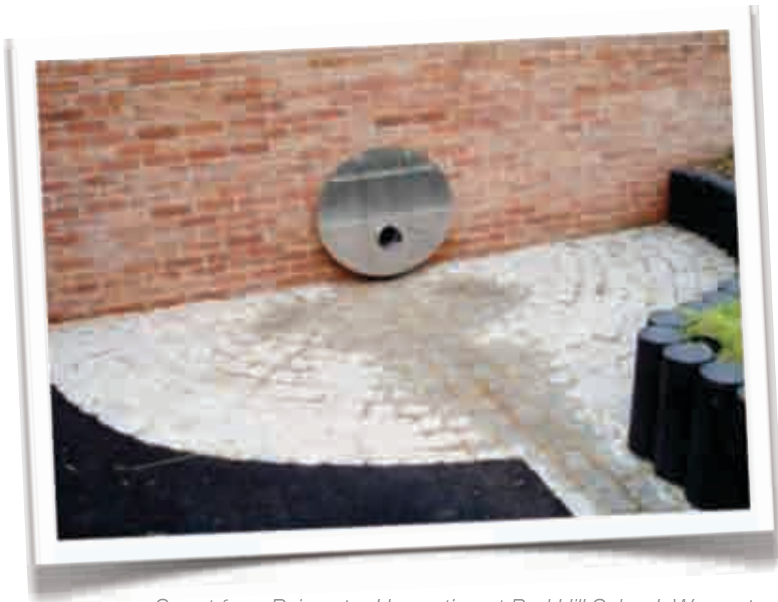
Spout from Rainwater Harvesting at Red Hill School, Worcester Image credit: Bob Bray Associates
