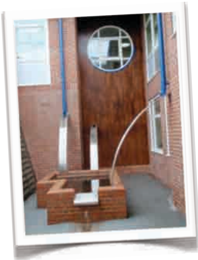
Collecting Runoff from Roofs at Fort Royal School, Worcester Image credit: Bob Bray
