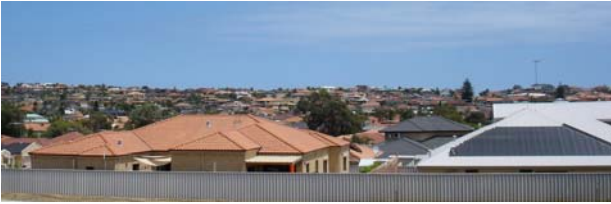
25 Spearwood WA, rear of houses. Note the narrow gap around the houses and the lack of windows
