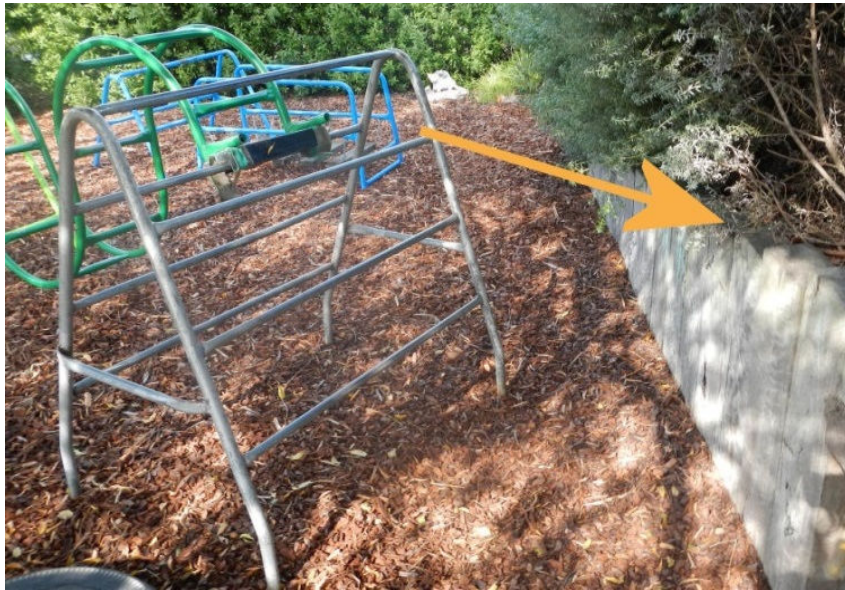
Too close to edging / wall
