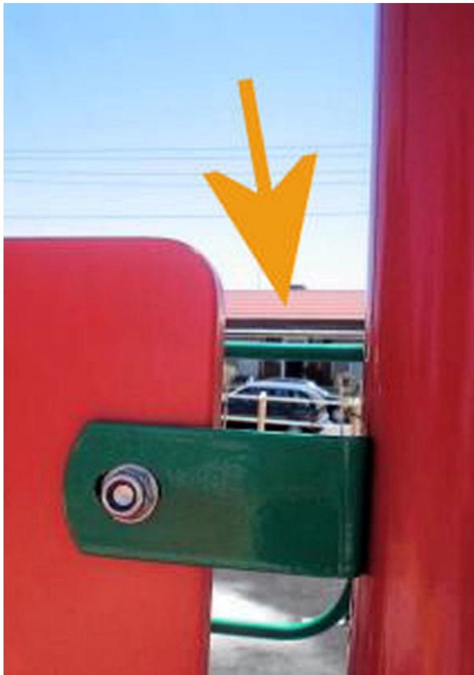
Gap at side of barrier and gaps between barrier slat tops are potential neck traps (>45mm wide and >45mm deep)
