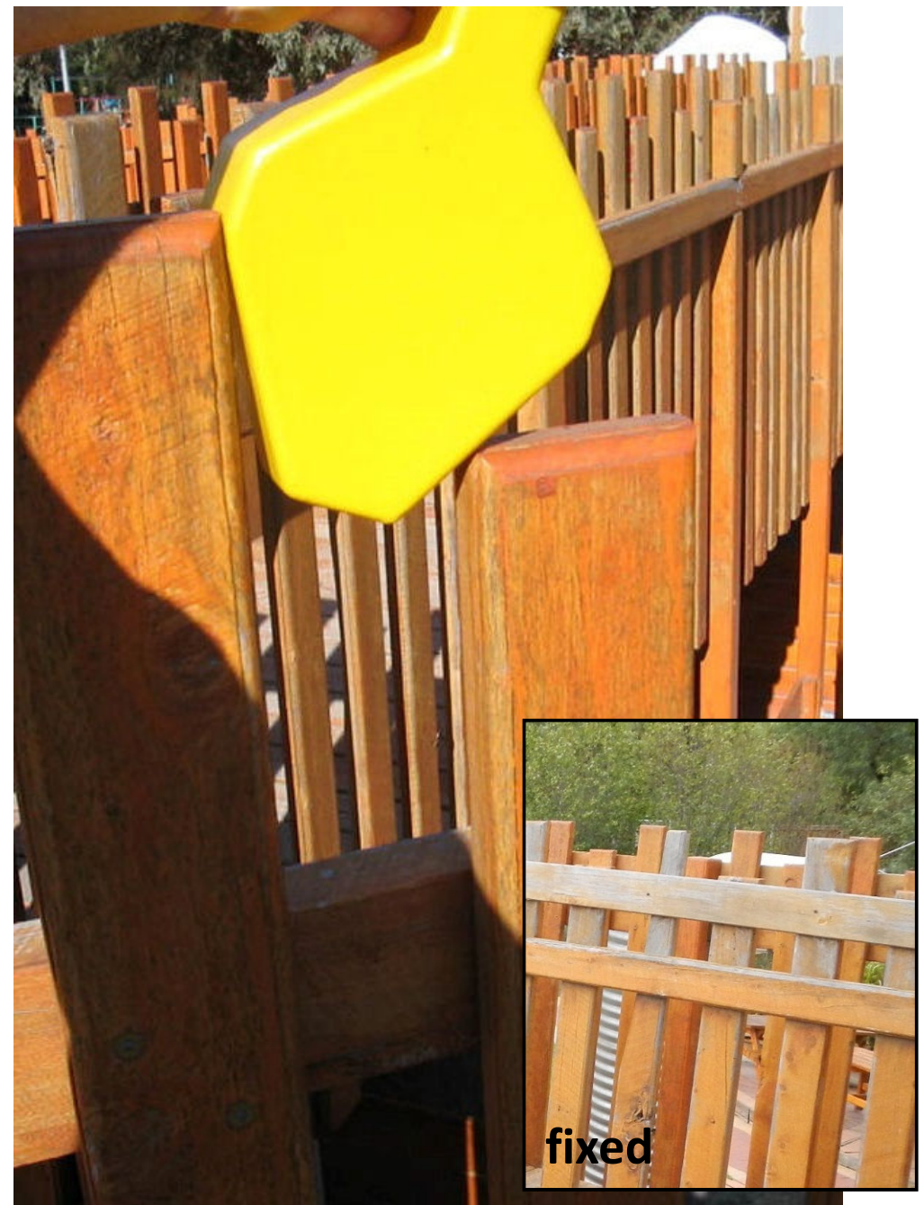
Gap at side of barrier and gaps between barrier slat tops are potential neck traps (>45mm wide and >45mm deep)
