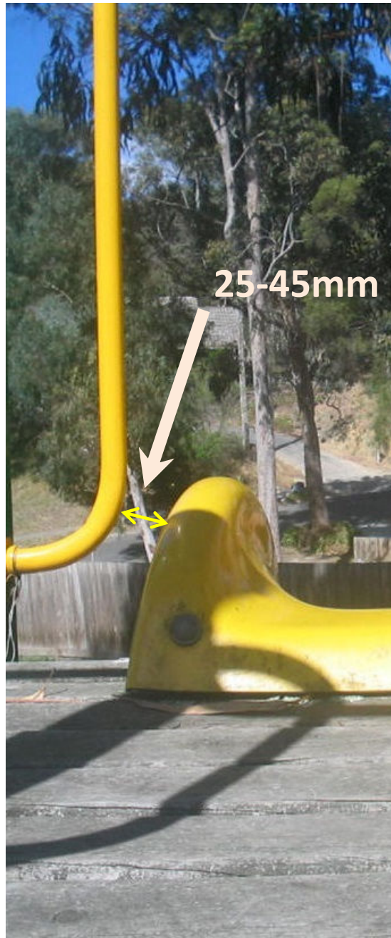
No potential neck traps at sides of slide by having gaps between 25-45mm
