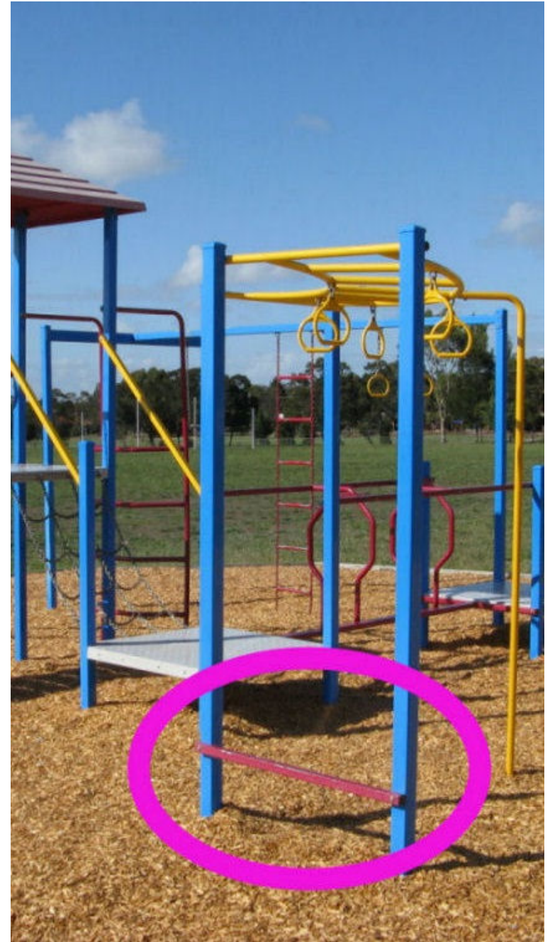
Horizontal rigid footbar at end of monkey bars could be a risk
