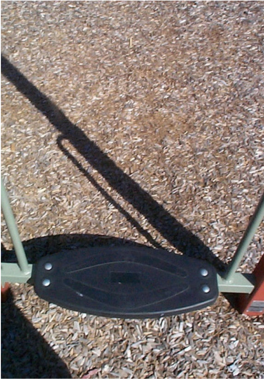
Wide rubber footpad at end of monkey bars is better than a bar
