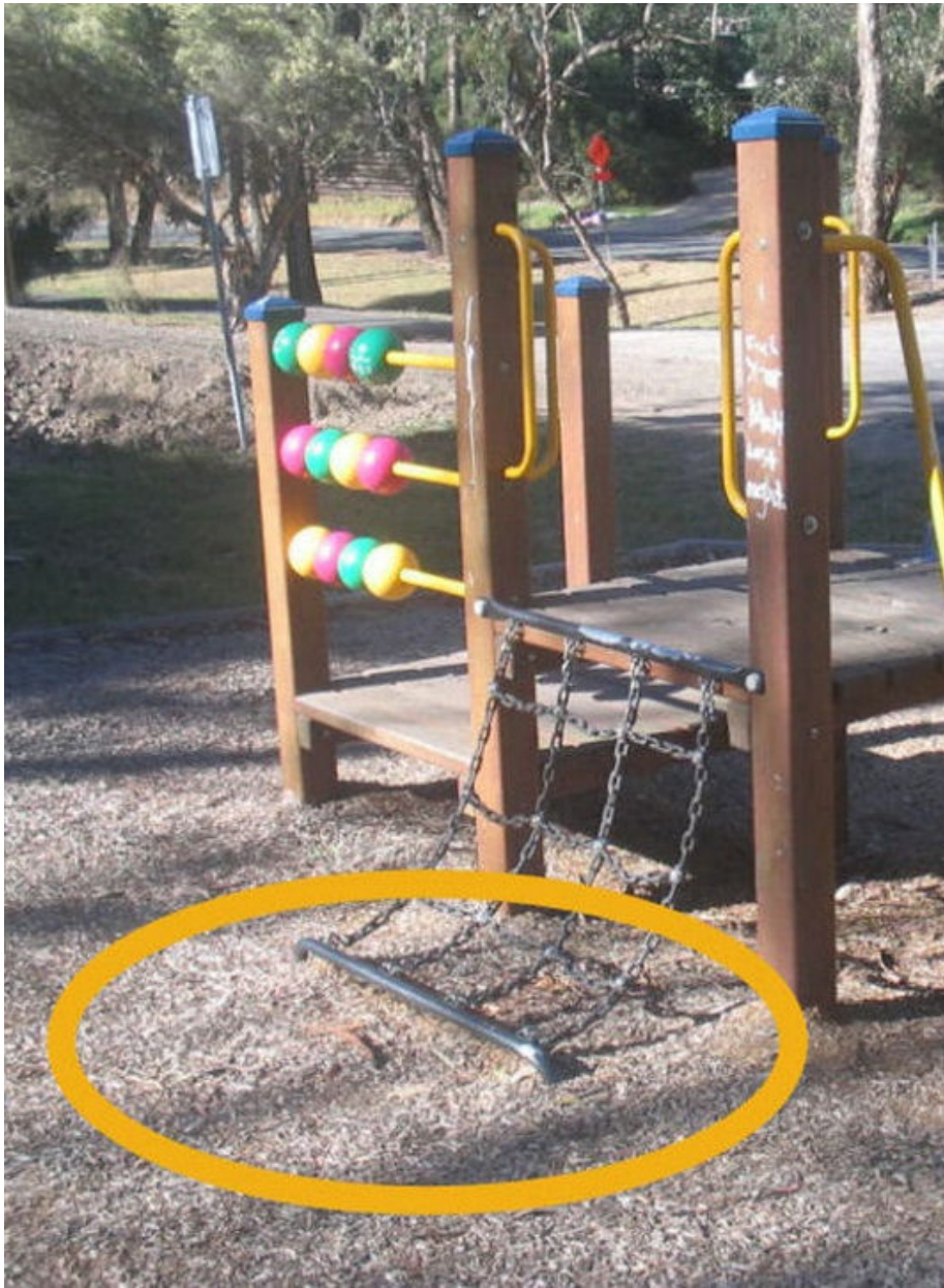
Exposed horizontal rigid bar at base of scramble net could be a risk
