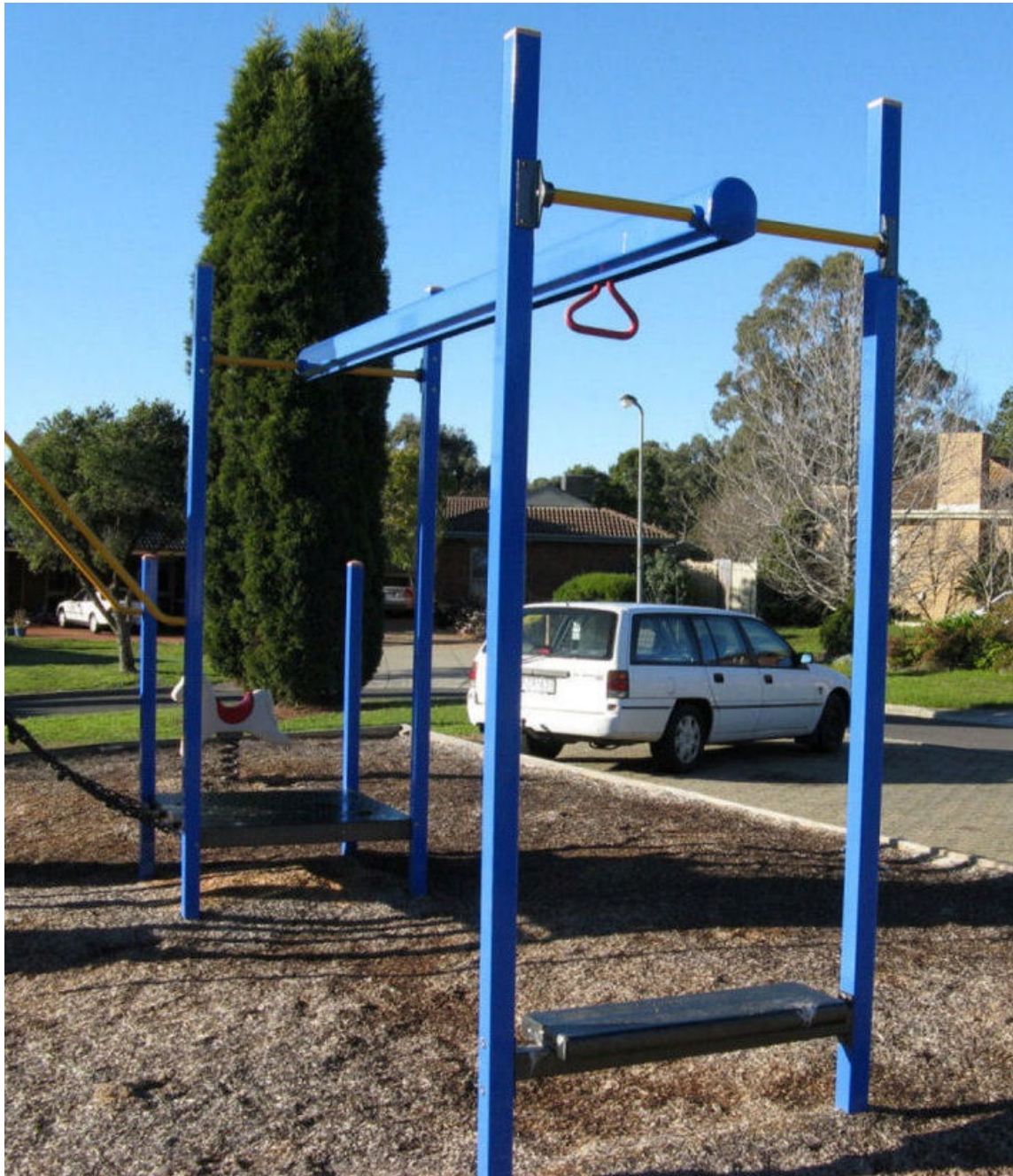
Small foot pad (and footbars) at end of track glide could be a risk – have nothing at one end at least
