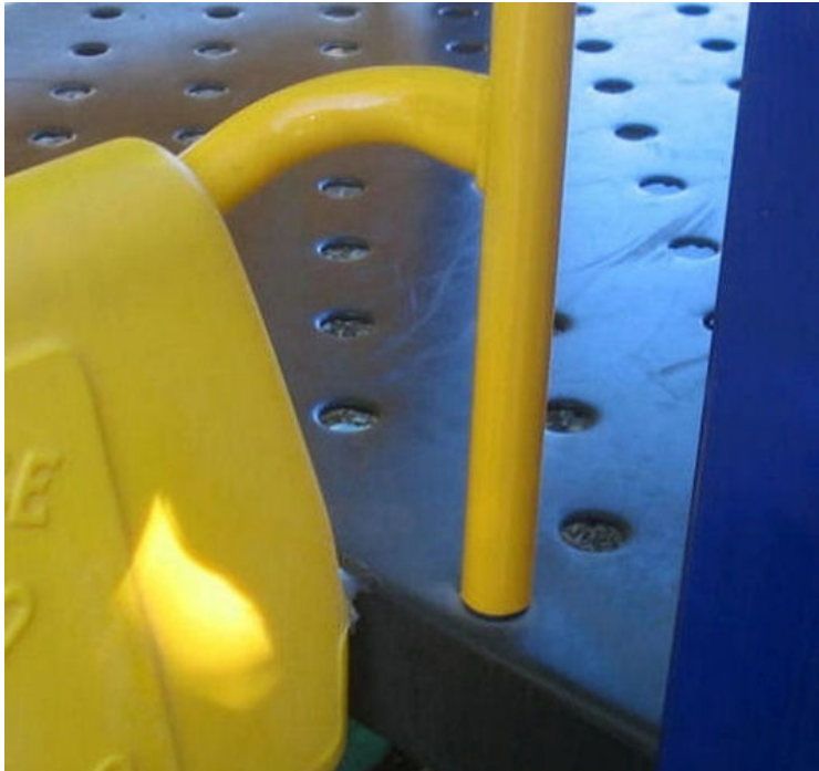
No potential neck traps at sides by having a bar across the top of the gap
