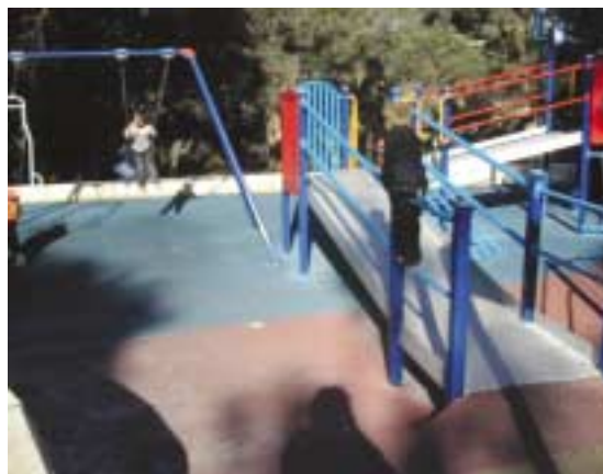
The orientation of the ramp prevents a child running across the swing fall zone
